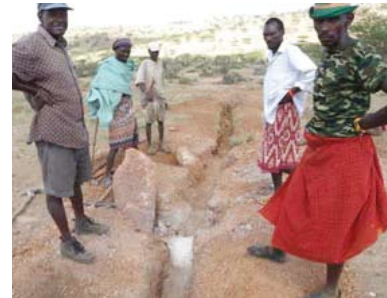
Digging trenches for pipes
